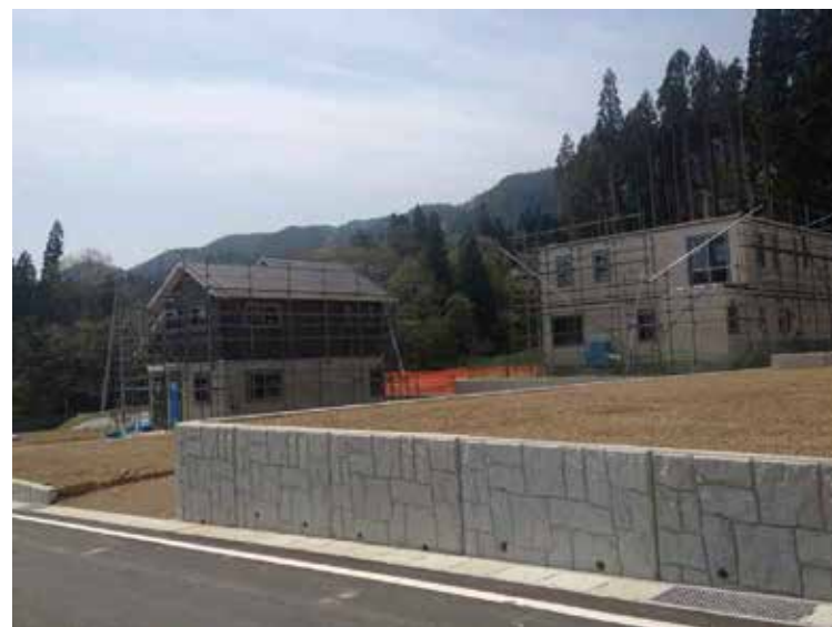
Housing construction has started
