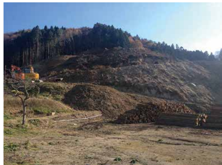
Cutting the sloping land for residential land use
