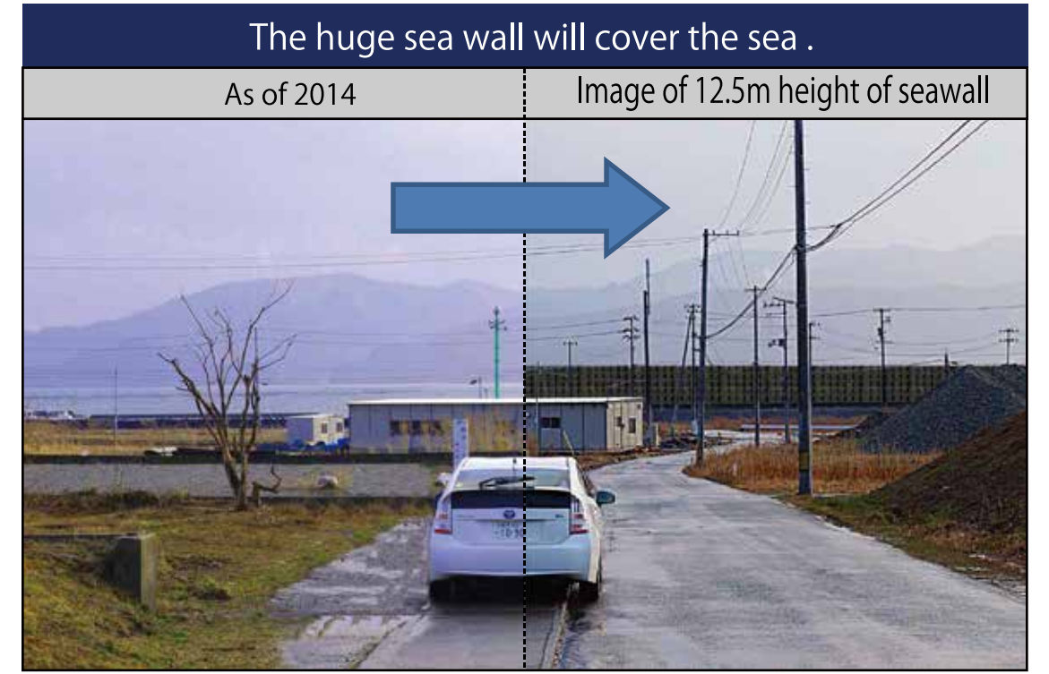
The view of Hirota bay of present and image of 12.5m height seawall
