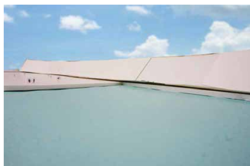
Model of a huge seawall, 12.5 m high
