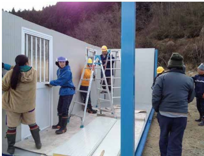
A scene of assembling the container by shop owners & volunteers
