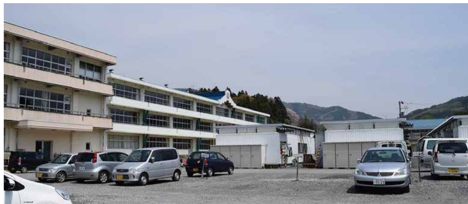
Temporary Houses Built in School Grounds
