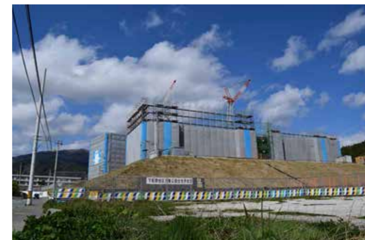
2014 Construction of public housing
